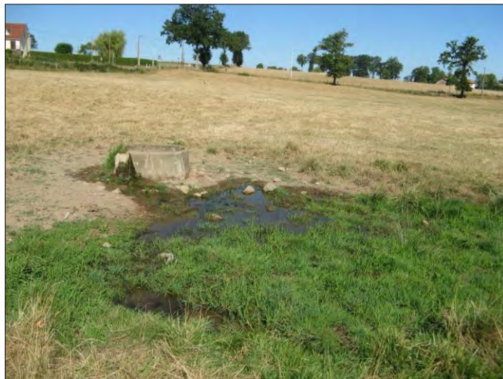
Photo 18 : îlot 22, captage buse béton
